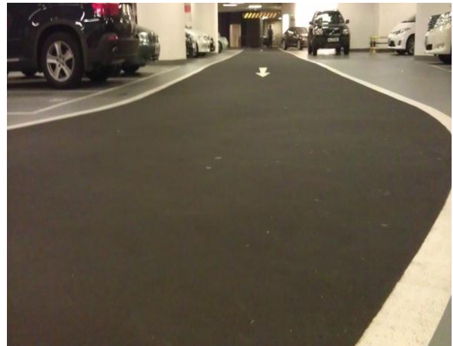
Nitoflor ET Slurry Application at a carpark in Hong Kong
