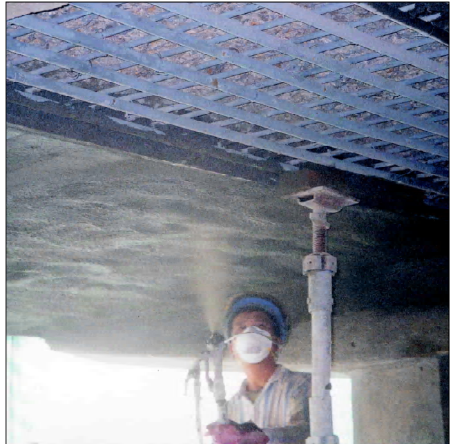
Sprayed repair project by Renderoc SPXtra for bridge deck soffit.
