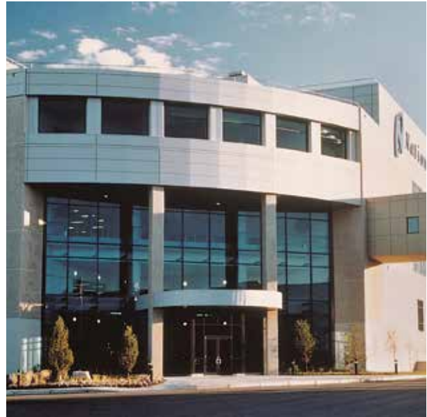
National Semiconductor Facility, South Portland, Maine, USA
