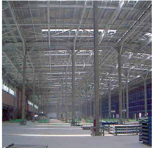
Korean Airlines Cargo Terminal, Incheon International Airport, Incheon, S. Korea
